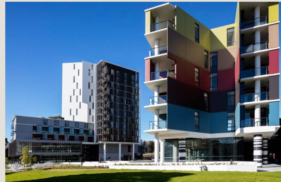
Taubmans Armawall Armashield coats the fibre cement sheeting and precast concrete external walls to ensure long-term durability, while cladding and balcony blades on the Epsom Road building are finished in Taubmans All Weather Low Sheen water-based paint – both feature dirt-shedding technology.
